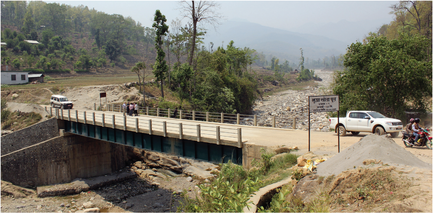
Vehicles on the newly constructed Jhupra Bridge in Surkhet and an NPTF monitoring team observing the construction.
